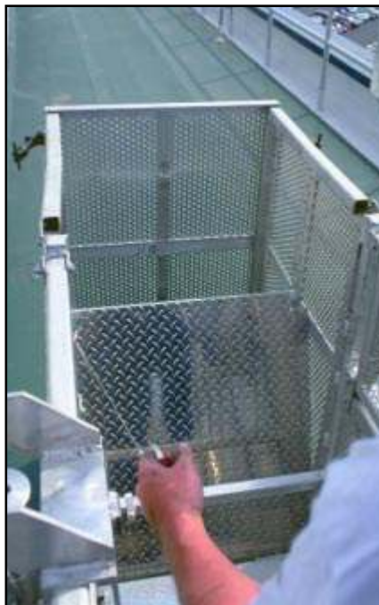
Extendable accordion-type tip out end is engaged for added reach before roof rigging this custom platform.
