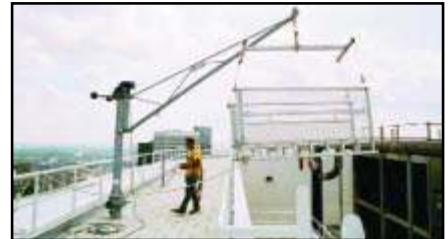
The platforms are suspended from trolleys mounted inside monorails located on soffit overhangs at the uppermost level of the buildings. Recessed balconies or building faces at the upper levels require platforms to be switched from an interior monorail to an exterior monorail and vice versa using a "turntable." To avoid using a perimeter-type electrical bus bar system of providing power to the platforms, battery powered trolleys are used at each platform "drop". The batteries are plugged into permanent electrical outlets located in soffits when not in use.
