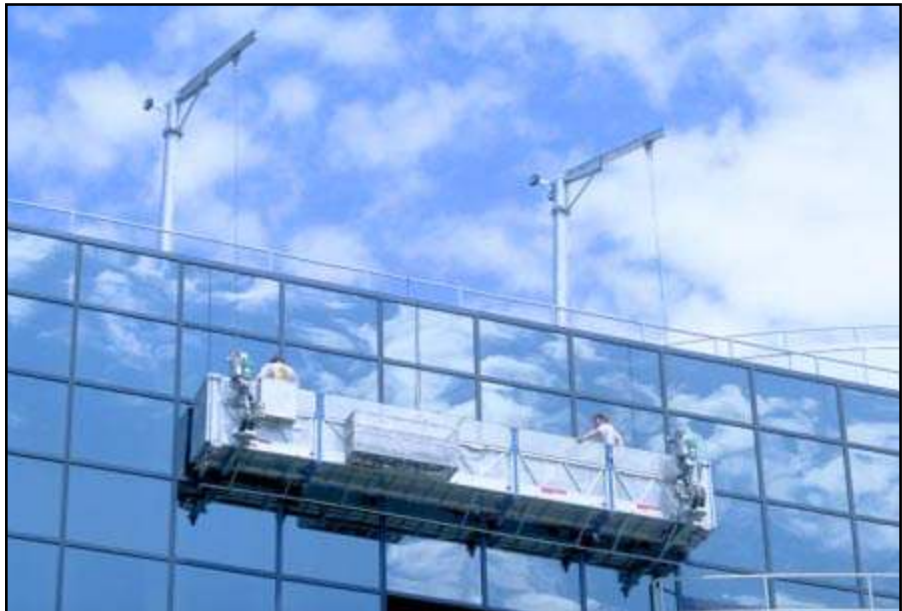
Permanent powered platforms are owner purchased and dedicated to a specific building. The Pro-Bel roof rigged system shown above (and on cover) is an F Type modular platform suspended from a Pro-Bel Davit System. See photos below. Bose Corporation, Boston, MA.
