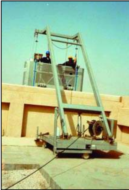
Pro-Bel Model PT 3008 Roof Car (Powered Trackless Trolley) is supported on hard rubber tired wheels and operates on a reinforced concrete bearing surface (or similar) cast on top of the roof finish. Steel base frame and suspension jib have 360° slewing and luffing (up and down) capability.
