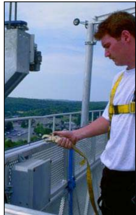
Four point suspension platforms include a permanently installed horizontal cable system (dog line) for the attachment of workers' fall arrest lanyards (no separate hanging lifelines).
