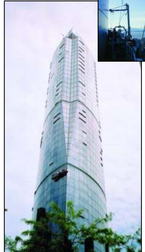
High-rise tower employs rolling davit carriage traveling on twin I-beam tracks at penthouse level. Modular platform can be reduced in size to service skylight notch. Inset shows davit carriage and loading area for platform. Wall Centre, Vancouver, British Columbia.
