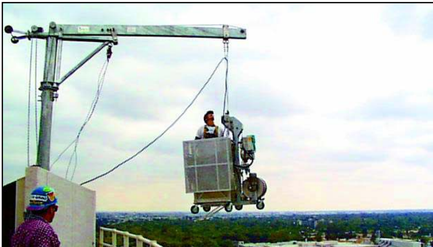
Pro-Bel single work cage is suspended from a Pro-Bel Tall Davit which is designed to clear the high parapet rail. Davit is equipped with two gear chains, one to facilitate arm rotation, and one to facilitate movement of rolling trolley inboard or outboard under load.
