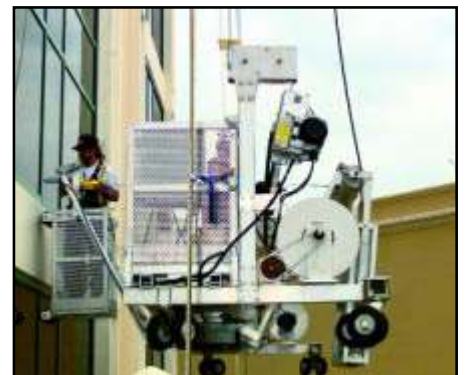
A heavy roller weight, located just above the electrical cable storage bin, counterbalances the cage in the outboard position while main suspension motor power is interrupted. Also, cage is designed to electrical-ly traverse sideways in tracks located below the main platform. Beau Rivage Hotel and Casino, Biloxi, Mississippi.
