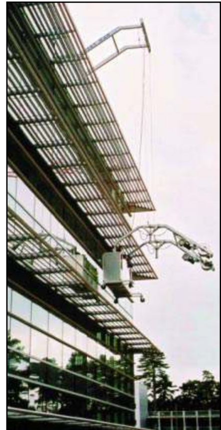
This platform utilizes a counterbalance or counterweight concept to help move the platform inboard of the suspension points which is very useful for reaching the glass under the sunscreens in this application. The platform moves laterally via a roof car thereby allowing convenient sideways movement controlled from the platform.
