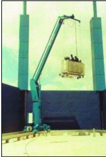
Pro-Bel Model RA 3006 Roof Car (Roof Anchored Trolley) is designed to clear very high parapets. Trolleys are supported on 4 wheel assemblies operating on galvanized track mounted on concrete piers cast into the roof slab. Steel base and suspension jib have 360° slewing and luffing (up and down) capability.
