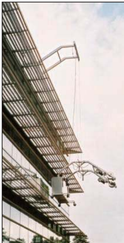
This roof car employs a counterweight to help move the platform inboard of suspension points to reach glass under sunscreens.
