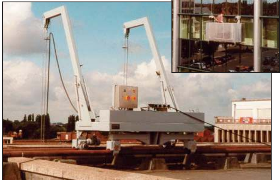
A variation of Pro-Bel Model FS-3000 Trolley Roof Car. Trolleys are supported on 4 wheel assemblies operating on galvanized pipe rails mounted on concrete piers cast into the roof slab. Steel base and suspension jibs have 360° slewing and luffing capability.
