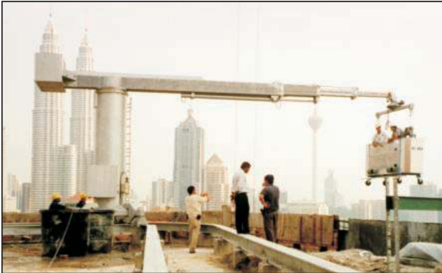
Pro-Bel Model RA T22 roof anchored trolley roof car with long single telescopic jib traveling on galvanized I-Beam track mounted on concrete piers. Slewing capability allows access to wide portion of building facade.
