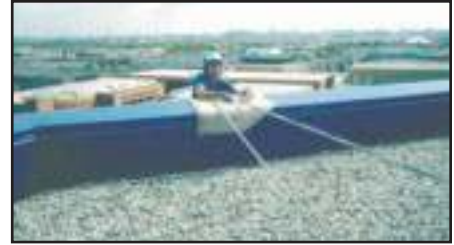
The chair is rigged directly to an anchor in line with the point of suspension. A separate independent anchor on the roof is required to secure the worker's fall arrest lifeline.
