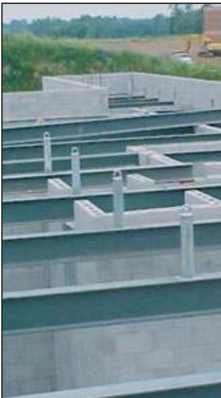
Pro-Bel roof anchors welded to beams before steel deck is installed.
