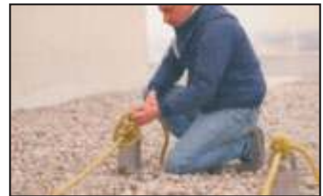
Pro-Bel safety anchors may be used for securing lifeline, for tie-back of primary rigging equipment or to directly rig a bosun's chair.
