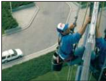
Bosun's chair is the equipment of choice among window cleaners. Pro-Bel safety anchors (see photo at right) are used to secure chair and separate lifeline.
