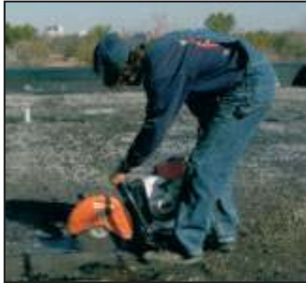
1. Small area of roof covering is removed down to concrete deck.
