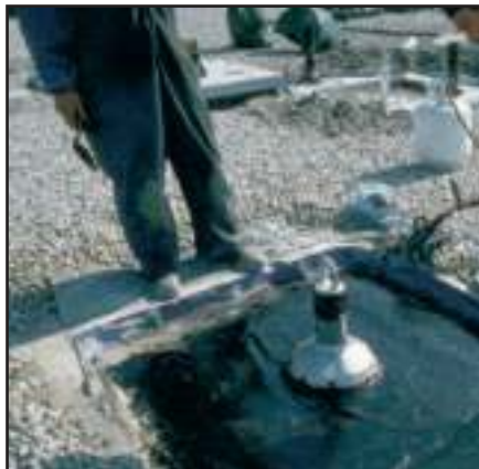
5. Top of spun aluminum flashing is sealed to steel anchor using a conformable mastic tape and heat-shrink rubber collar flashing.
