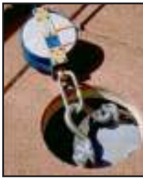
Anchor in terrace deck. Paver cutout conceals anchor when not in use.
