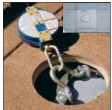
Pro-Bel “flip-up” terrace anchor concealed with cut out core trimmed with stainless steel band and tabs.
