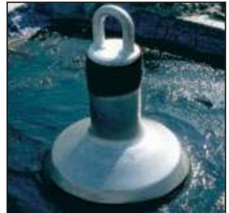
6. Close-up of anchor. Installation method is similar for both conventional roof (membrane above insulation) and protected membrane roof (membrane below insulation).
